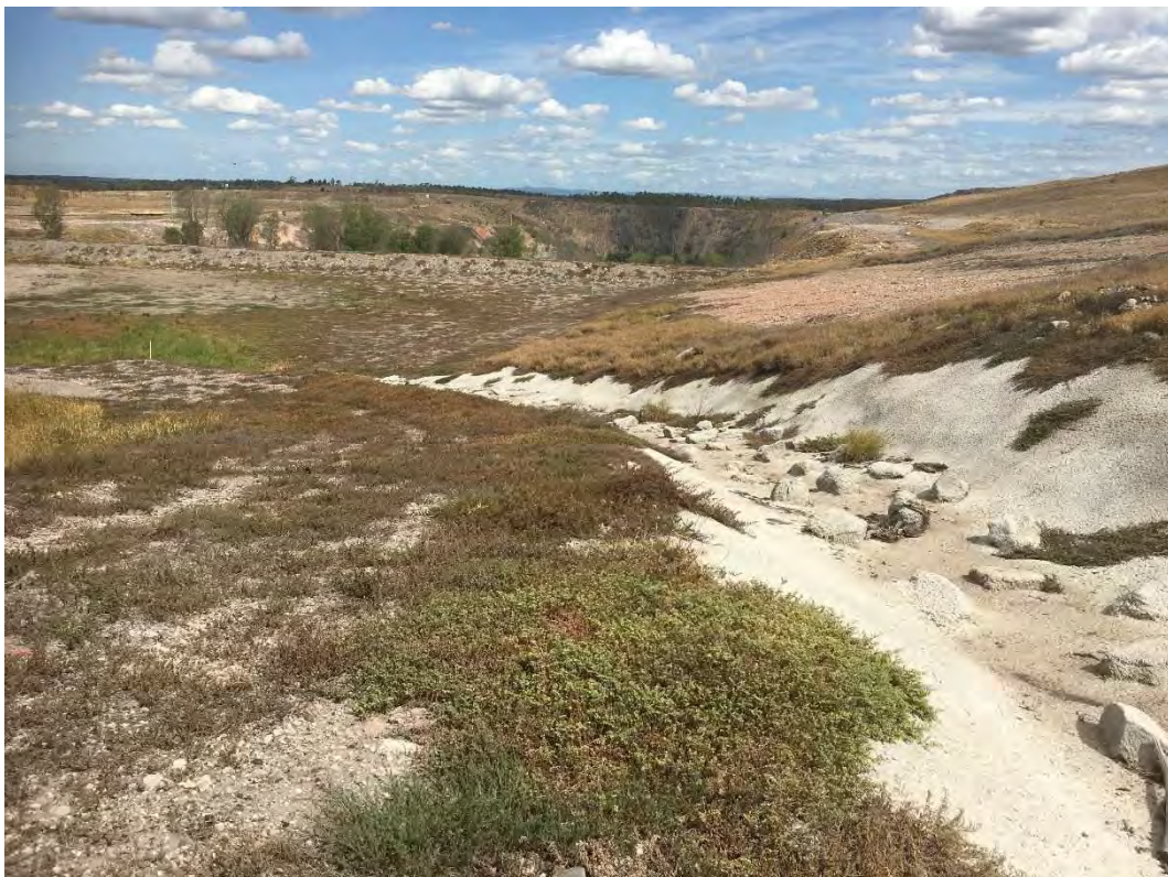
Rock lined spillway chute from Stage 1 compost pad to leachate dam
