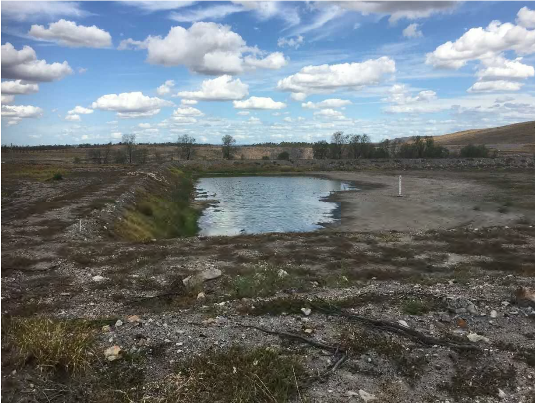
Leachate dam and spillway (middle of left embankment)
