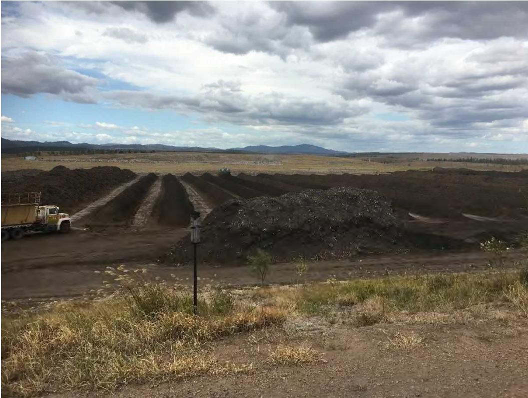
Existing compost pad (Stage 1)
