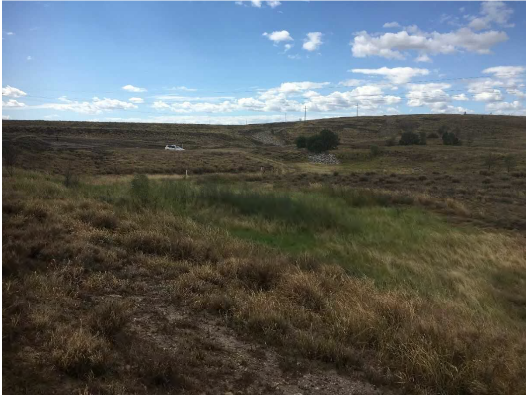
Clean water diversion spillway (background) through to lower basin (foreground)
